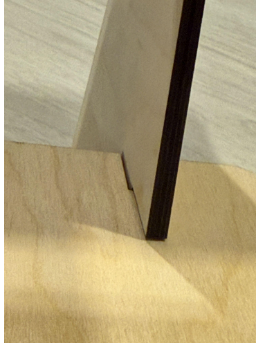
Figure 4.6: Close-up of gap/misalignment
